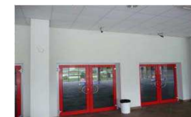
Window sticker on the west side of G pavilion
