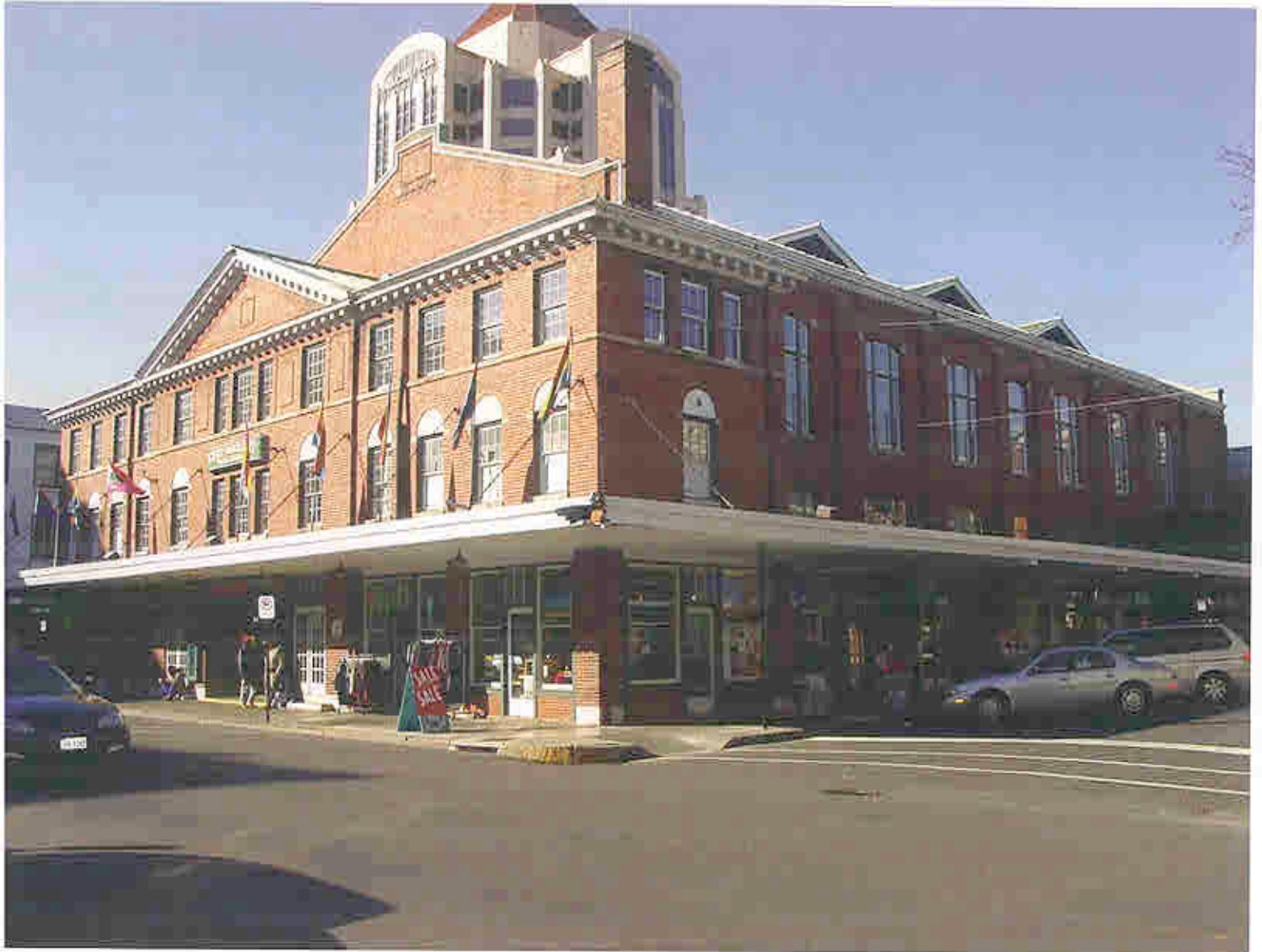
SOUTH AND EAST ELEVATIONS
