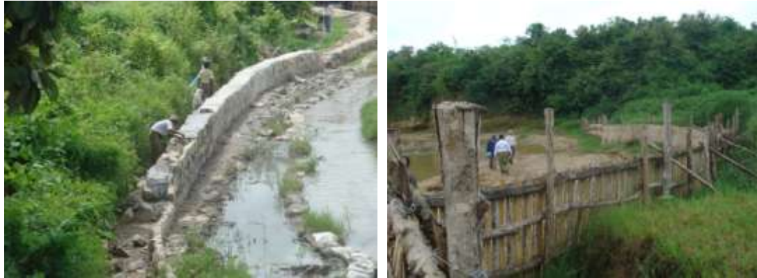
Stream bank protection structures in Myanmar. Left: Stone-cement structure, Right: Bamboo and wooden structure. Photographs by M. Dhakal
