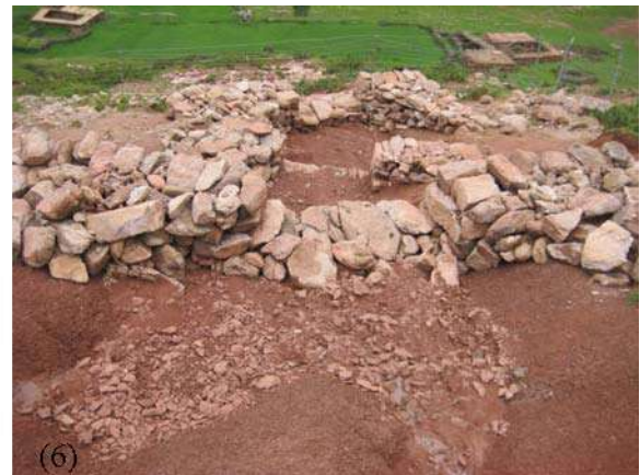
Photo (3) Gully before check dam construction, (4) local people involved in check dam construction, (5) and (6) a series of 3 check dams (after completion)
