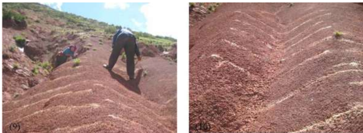
Photo (9) and (10) Grass seed sowing in diagonal line
