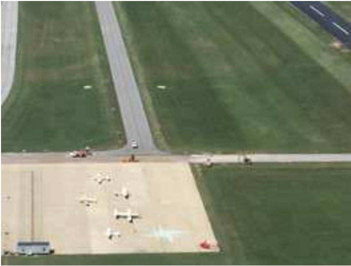
construction at Taxiway Bravo and the ramp
