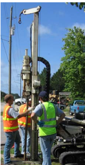
Drilling a micro well using Direct Push Technology
