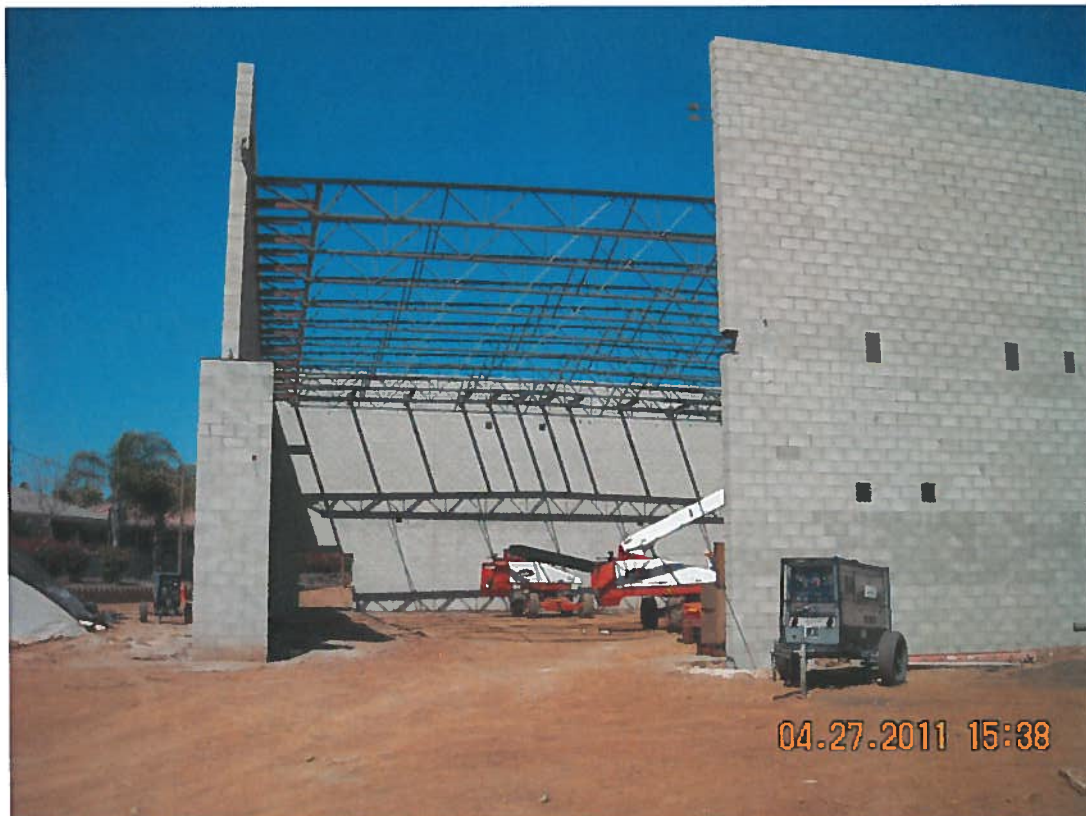
TRUSSES AT BUILDING 'A'
