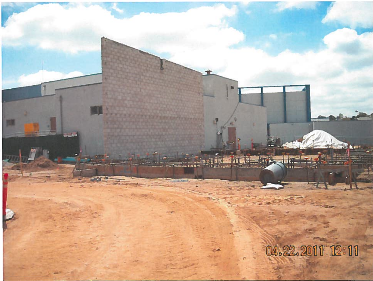
CMU WALL AT THE PAC
