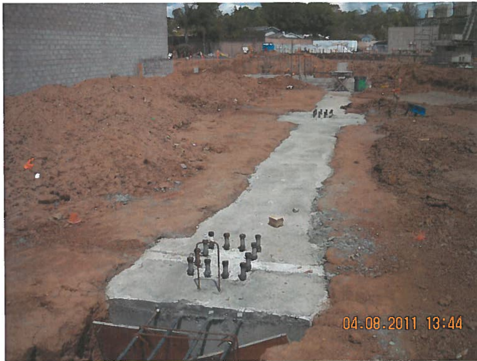
GRADE BEAM AT BUILDING A DANCE
