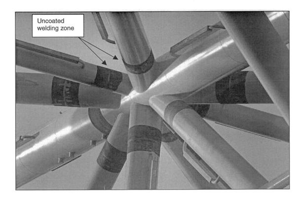
Figure 1 – Intersection between bracings and legs
