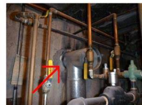
Heater in enclosed rm, furnace cement
