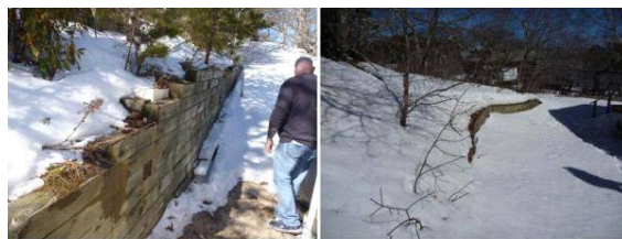
Retaining walls, PT wall greater than 4 ft
