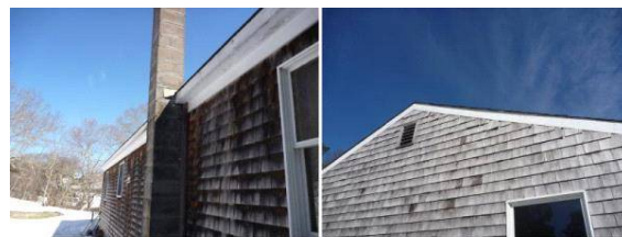
Aged at rear, loose at rake board
