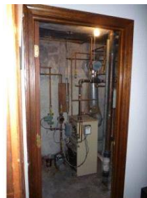
Heater in enclosed rm, furnace cement
