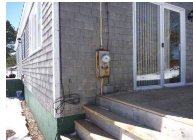
Meter box rusted.
