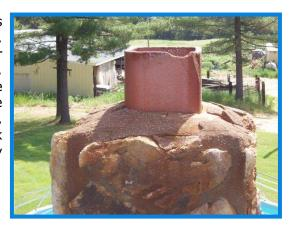
**REPAIR NEEDED:** The chimney(s) requires repairs, specifically in the form of tuckpointing cracks in the masonry stonework.
