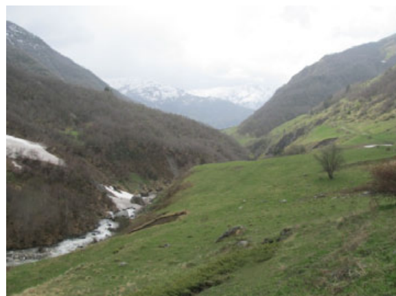
The dam at the Khaldestchala River. Image taken by HIPP team during the field visit
