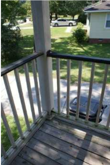
Hand rails are loose or rotted at the attachment points. This is a dangerous situation because someone might lean against them and fall.
