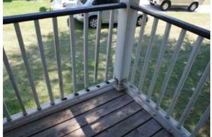
Hand rails are loose or rotted at the attachment points. This is a dangerous situation because someone might lean against them and fall.
