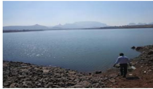
River Godavari at Kashyapi Dam
