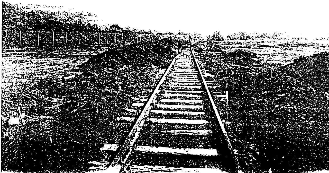
Fig. 4. Railroad tracks at the former ore storage site in Palmerton, Pennsylvania (PP001), looking east (August 1988). Piles of soil and debris were moved to allow access to the area around the tracks.
