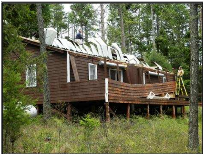
Before: Hi-Line cabin - April 2013
