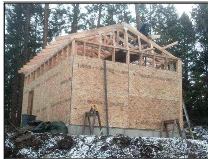
New pump house - February 2014
