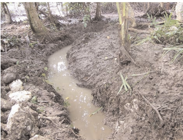
Volunteers from Radefasu, in Malaita Province, work together to build a drainage system (top) and the results of their efforts (above).
