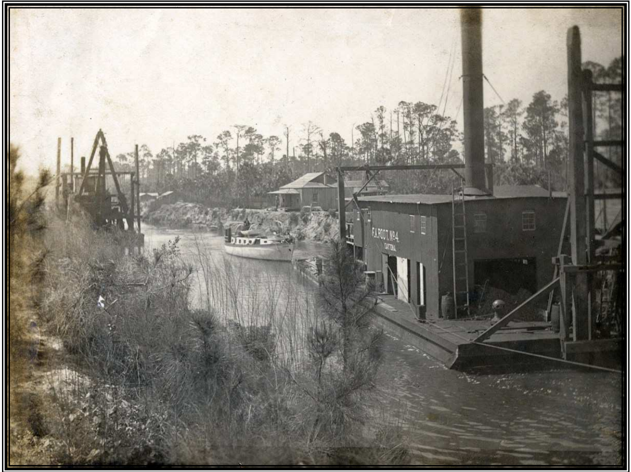
Dredging of the Intracoastal Waterway Canal in Palm Valley. (1916)
