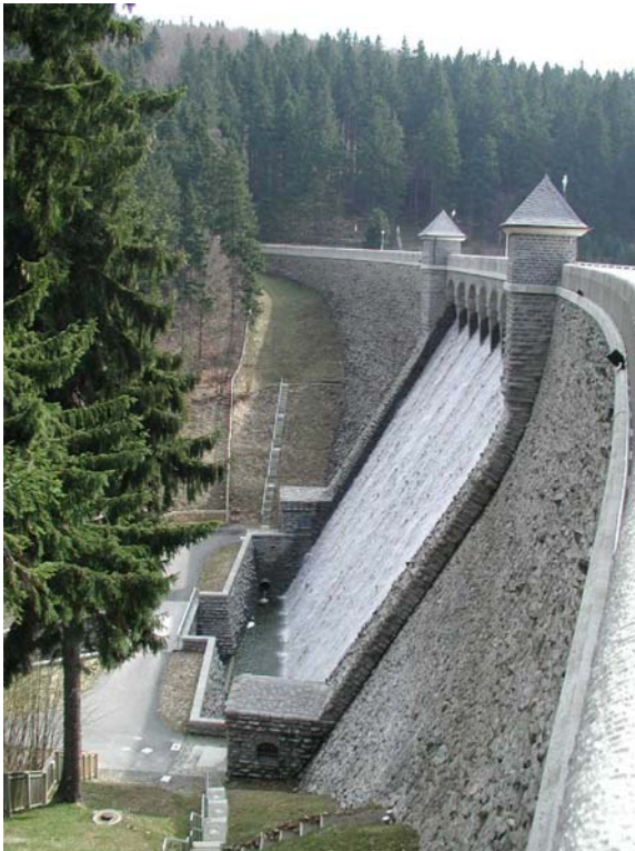
Fig. 6 Downstream view with spillway
