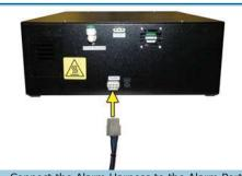
• Connect the Alarm Harness to the Alarm Port on the back of the Dehydrator.
