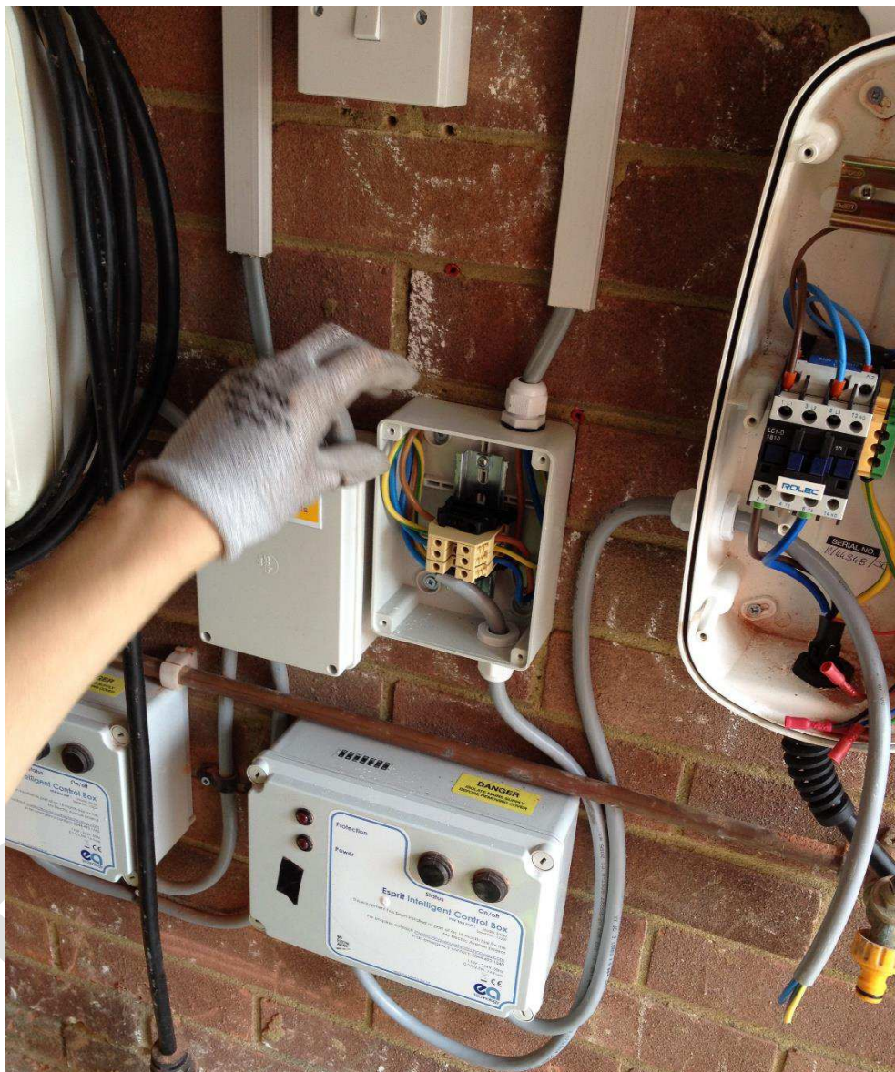
Figure 4. Example photograph of connected terminal box.
