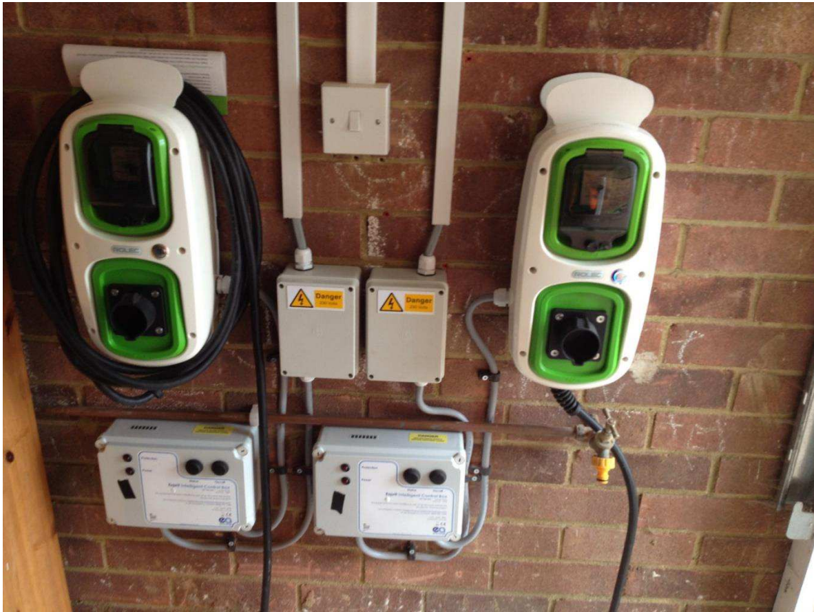
Figure 5. Example photograph showing the location of the charging point, ICB and terminal box.
