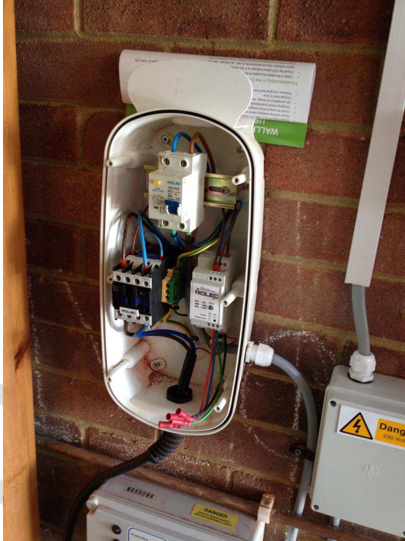
Figure 3. Example photograph of connected charge point.
