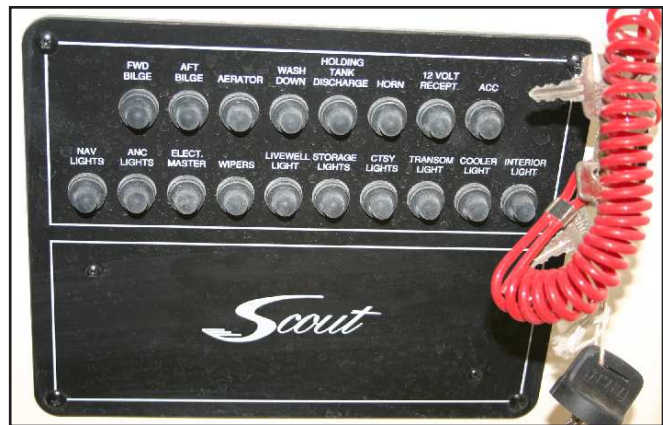
Helm Circuit Breaker Panel Below Steering Wheel
