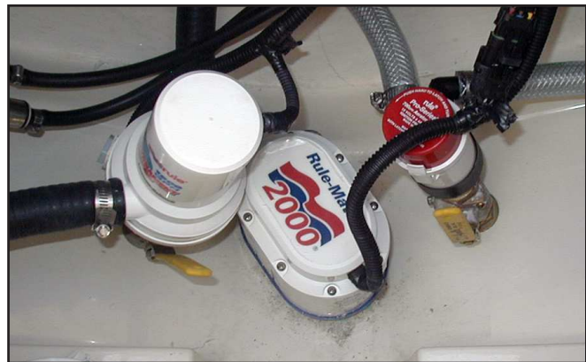
Livewell and Bilge Pumps in Stern Bilge
