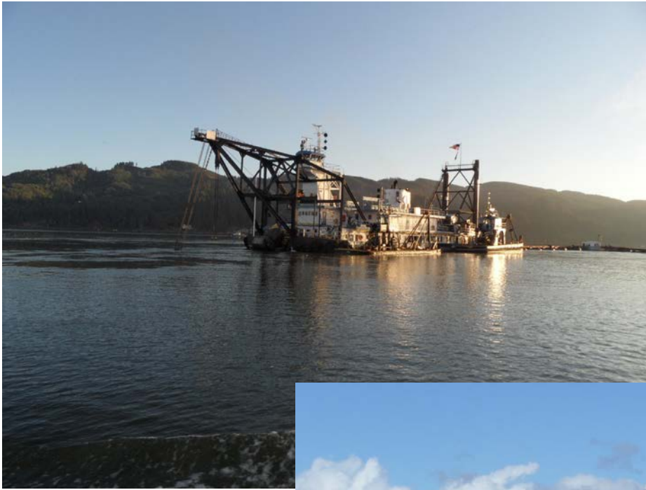
Photos of pipeline Dredge Oregon
