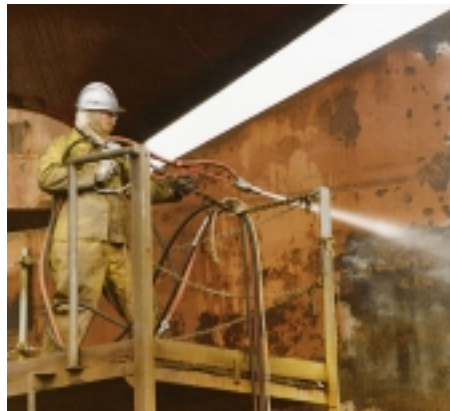
High Pressure Wet-Blasting System
