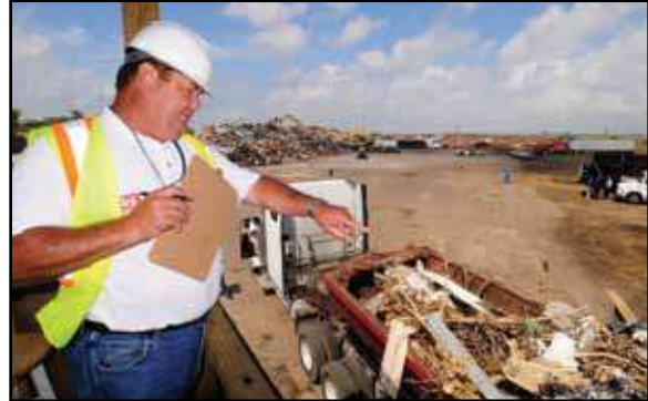
Figure 6: Debris monitors determine type and quantity of debris
