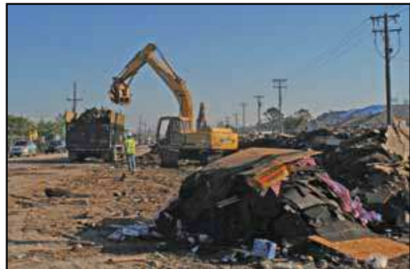
Figure 1: Contractor debris operation
