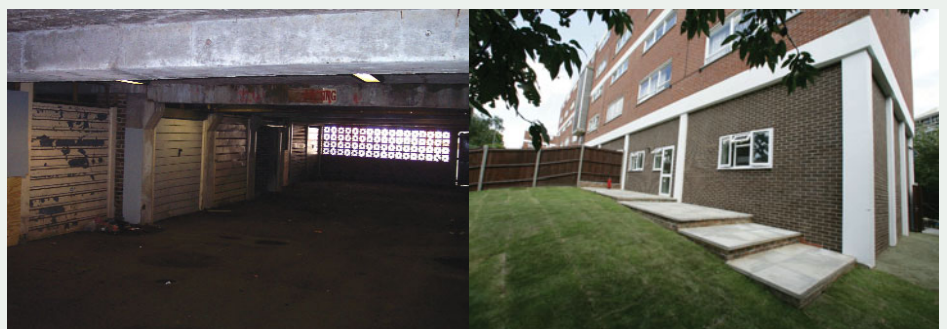
Hidden homes – before and after
