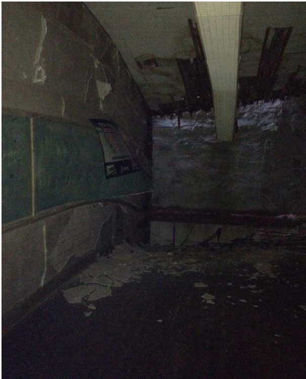
8 Second floor northwest classroom where roof and wall collapsed.
