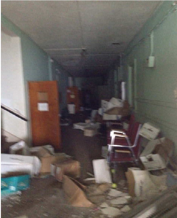
First floor corridor
