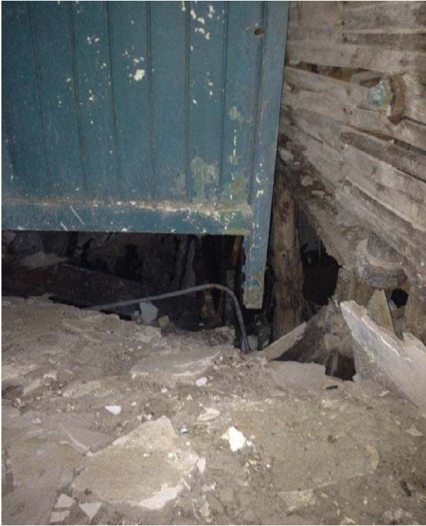
10 Second floor northwest classroom where roof and wall collapsed.
