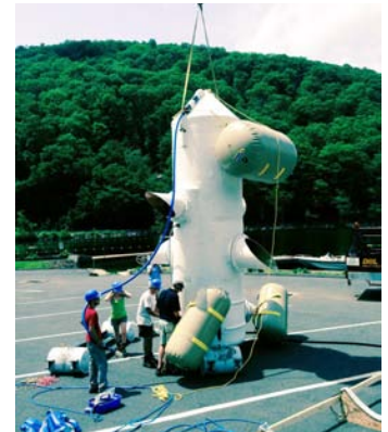
Pontoons were attached to the Systems to allow them to be floated and towed to installation points off Arrowpoint.
