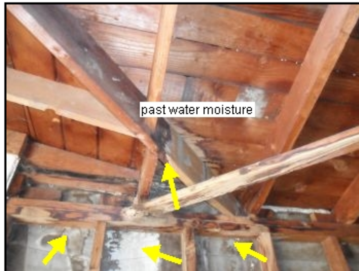
Garage Roof Condition
