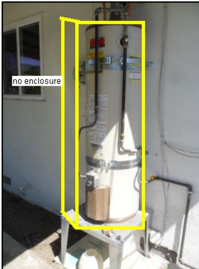
Water Heater Heater Enclosure
