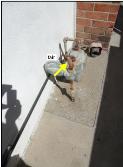
Grounds Main Gas Valve Condition
