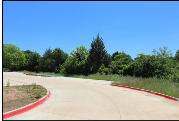
View C: View to the east property line
