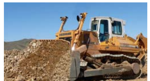
PR-752 in Boroo Gold mine site
