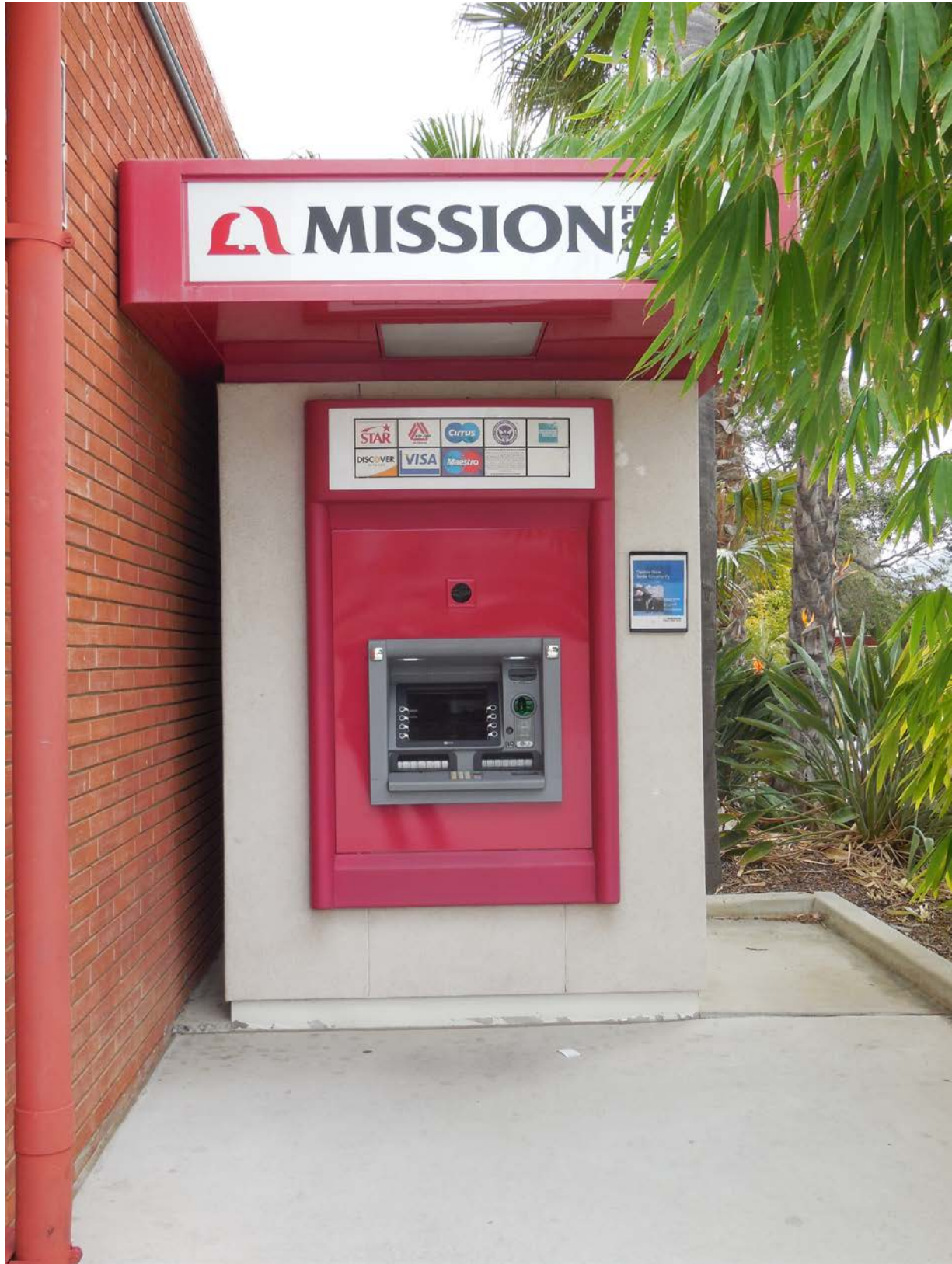
Front of ATM Structure
