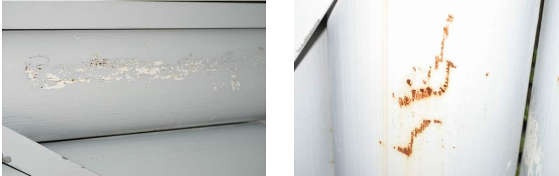
Figure 5.1 Corrosion
