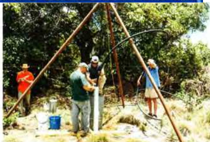
Lance trying to access ground water using the Baptist well drilling method
