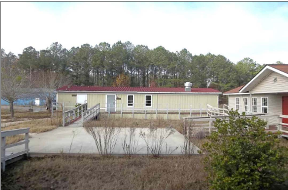
Kitchen/Dining Room Building Improvements
