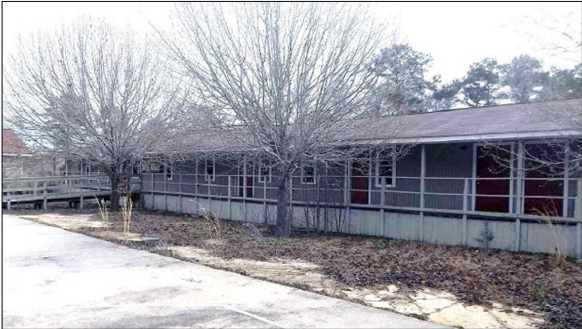
Classroom Building Improvements
