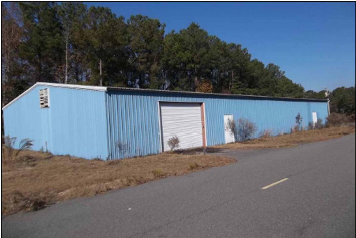
Storage Building Improvements
