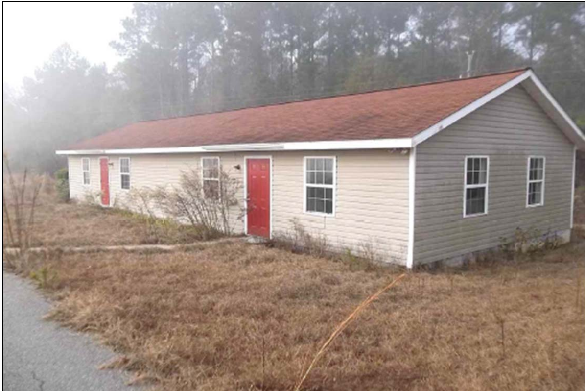
Classroom Building Improvements
