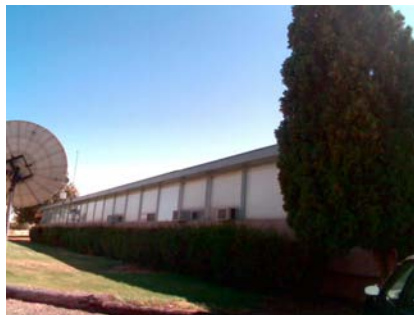
NE Elevation View
