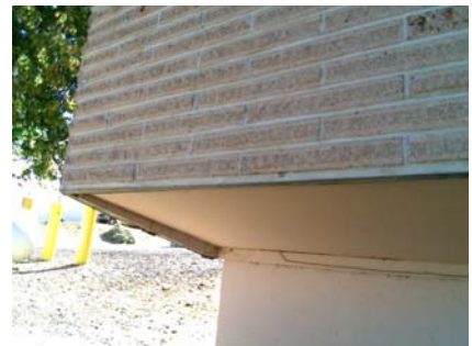
NE Primary Structural Type WOOD SIDING BENEATH BRICK
