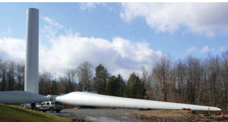
When standing in front of a wind turbine, its impressive size is striking.
