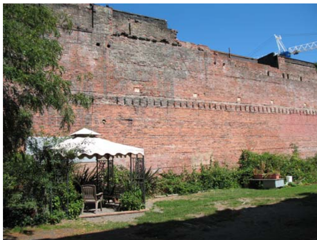
Figure 7: The site is used by the community for various social gatherings, and as a garden and sitting area for the adjacent cafe.
