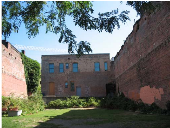
Figure 6: Case Study site: this site is void of built structures. The remaining elements of the original building are a fire door next to the easement at the rear of the lot, and party walls still used by adjacent buildings.
