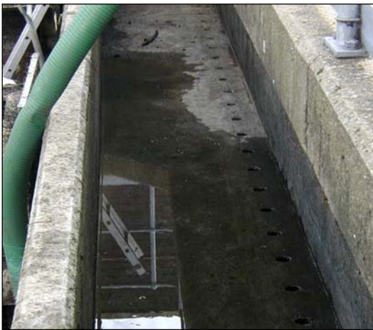
Figure 4.4 A Primary filter bed inlet at Coppermills WTW, North London before an influx of mussels.
