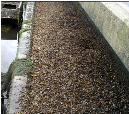
Figure 4.5 The same filter bed inlet as in Figure 4.4, after an influx of mussels.
