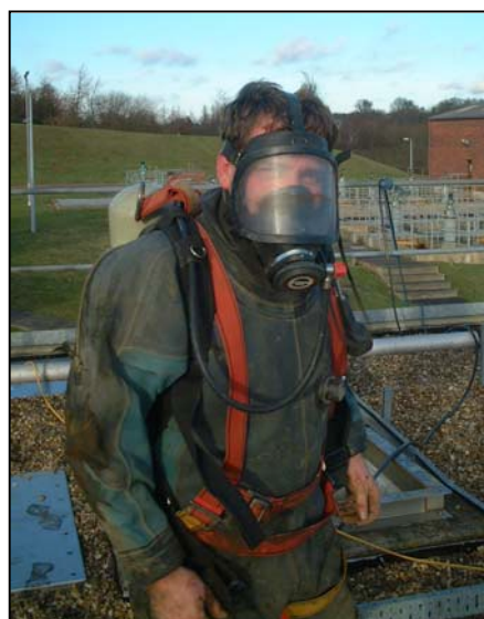
Figure 4.10 Protective equipment used to clean mussels from ozone tanks at Alton WTW, Suffolk.
