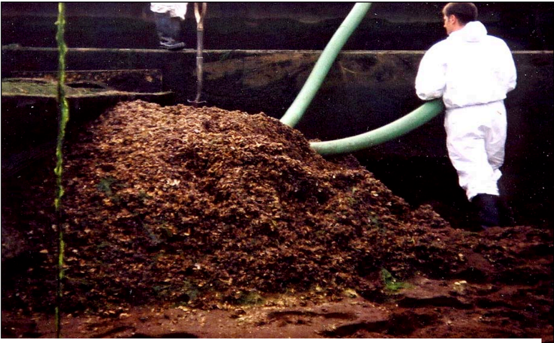
Figure 4.6 Mussel shells in a primary filtration bed at Coppermills WTW (October 2001).
