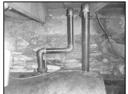
After: piping is black iron and of proper size
