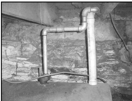
Below: Piping is plastic and too small for the job!
