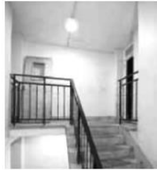
photo of stairwell with LED fitting
