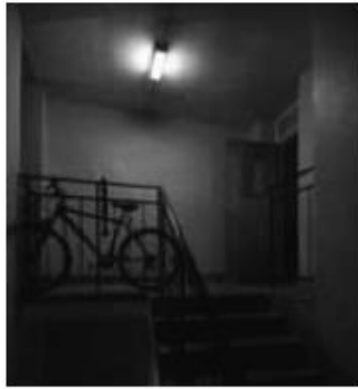
photo of stairwell with fluorescent fitting
