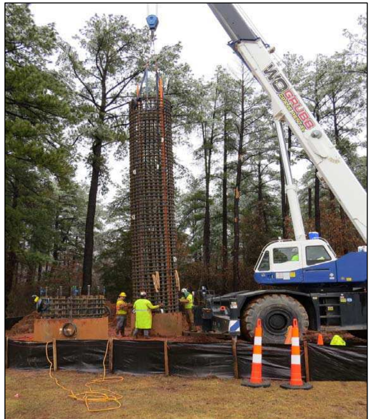
Once in the ground, concrete will be poured around these rebar cages that will reinforce the test shafts. Photo by: Chuck Samuelson, MWAA
