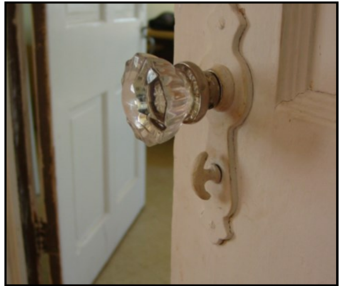
Original Glass Doorknob in the Historic Caretaker's Home
