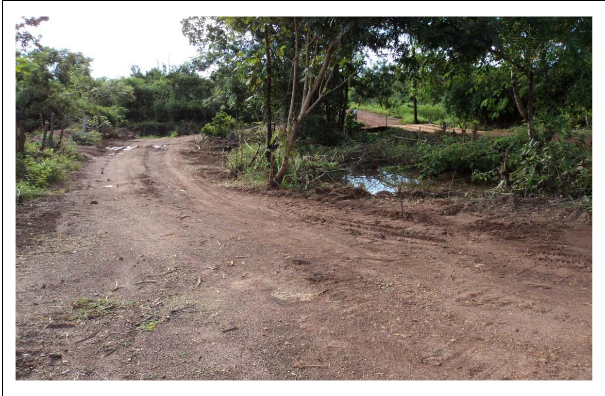
Constructed Diversion Road at R213 PK 1+852 (Preah Vihear)
