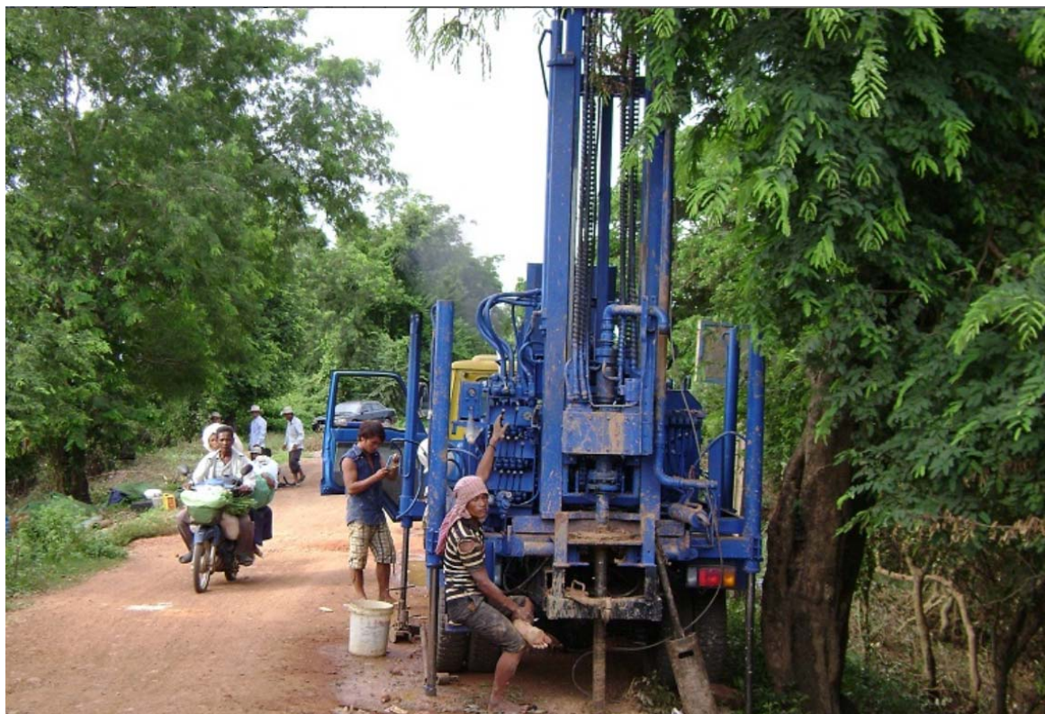
Foundation Investigation for the Proposed Bridge at PR207
