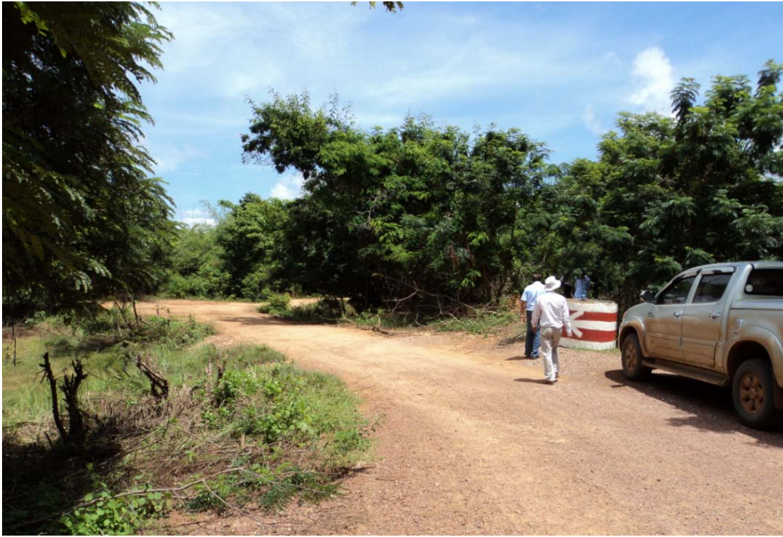
Existing Diversion Road for Proposed Bridge at PK 2+ 670 PR18-1 (Oddar Meanchey)
