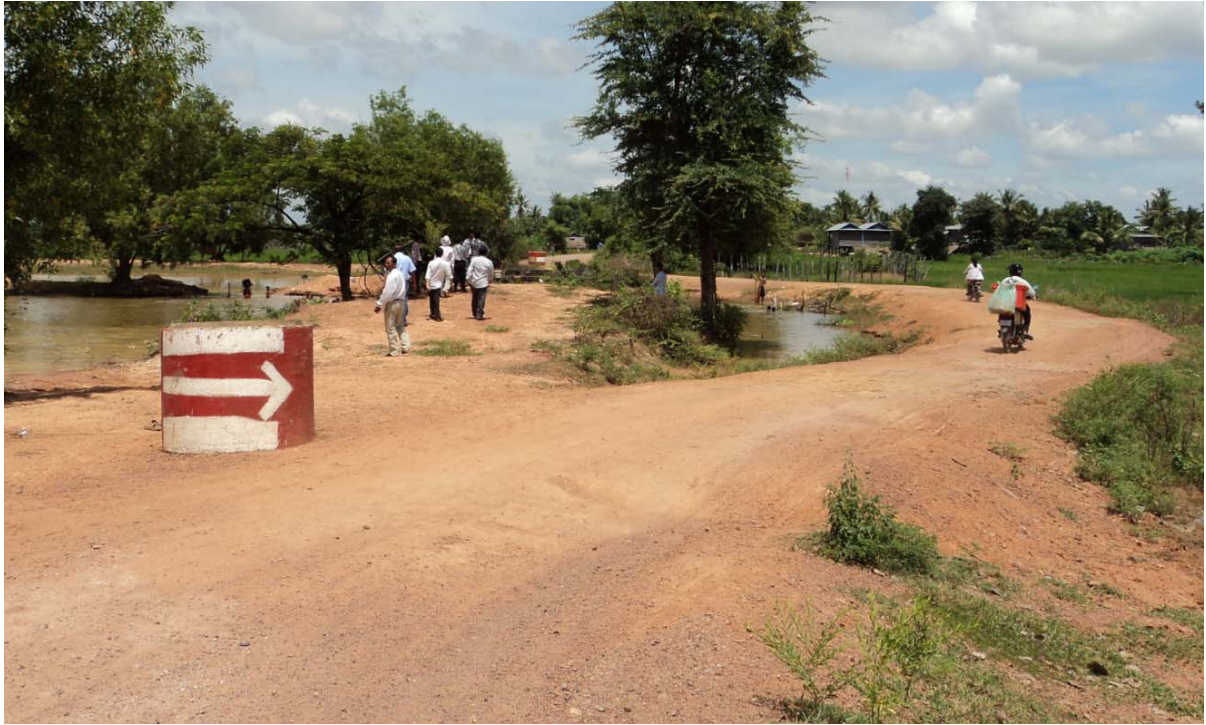
Existing Diversion Road for RC Box Culvert at PK 5+ 440 PR181-1 (Oddar Meanchey)
