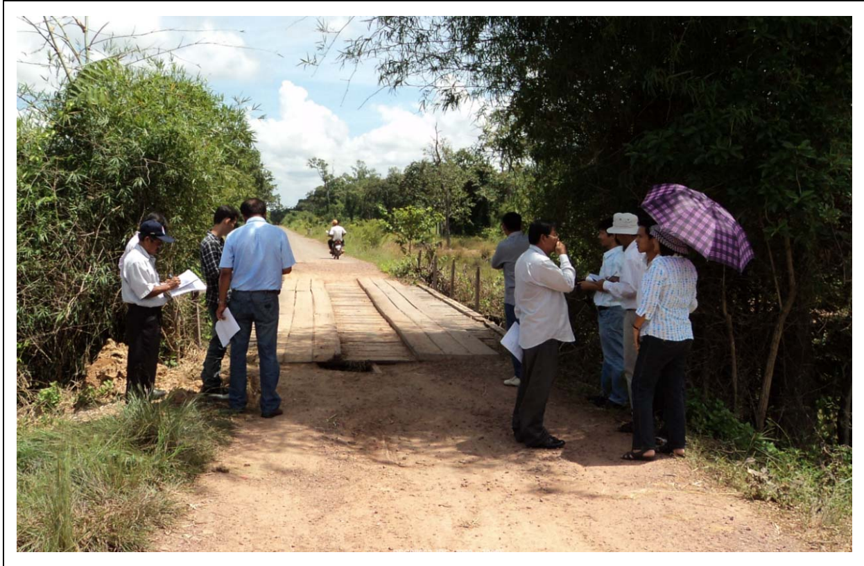
Existing Wooden Bridge at PR181-1 PK 12+ 190 (Oddar Meanchey)
