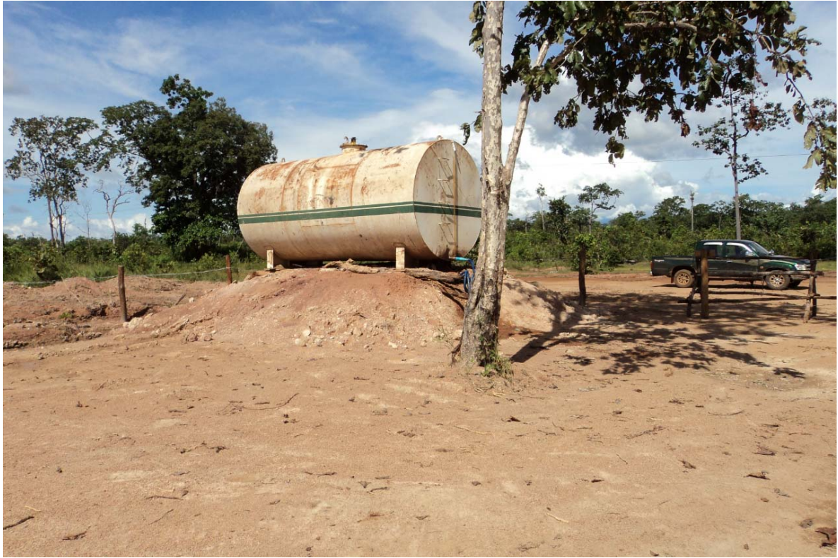
Typical Contractor's Fuel Depot at R213 Creating Environmental Concerns from WB Mission
