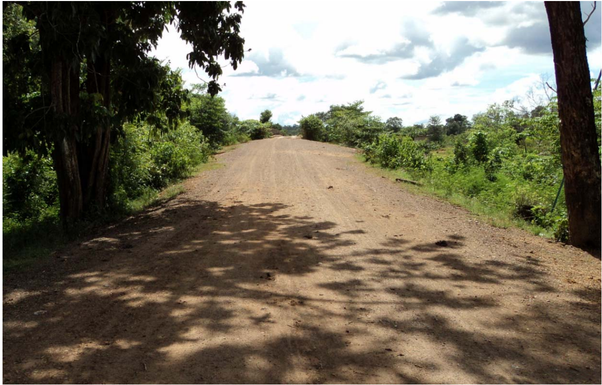
Project Road R213: Existing Road Section and Condition
