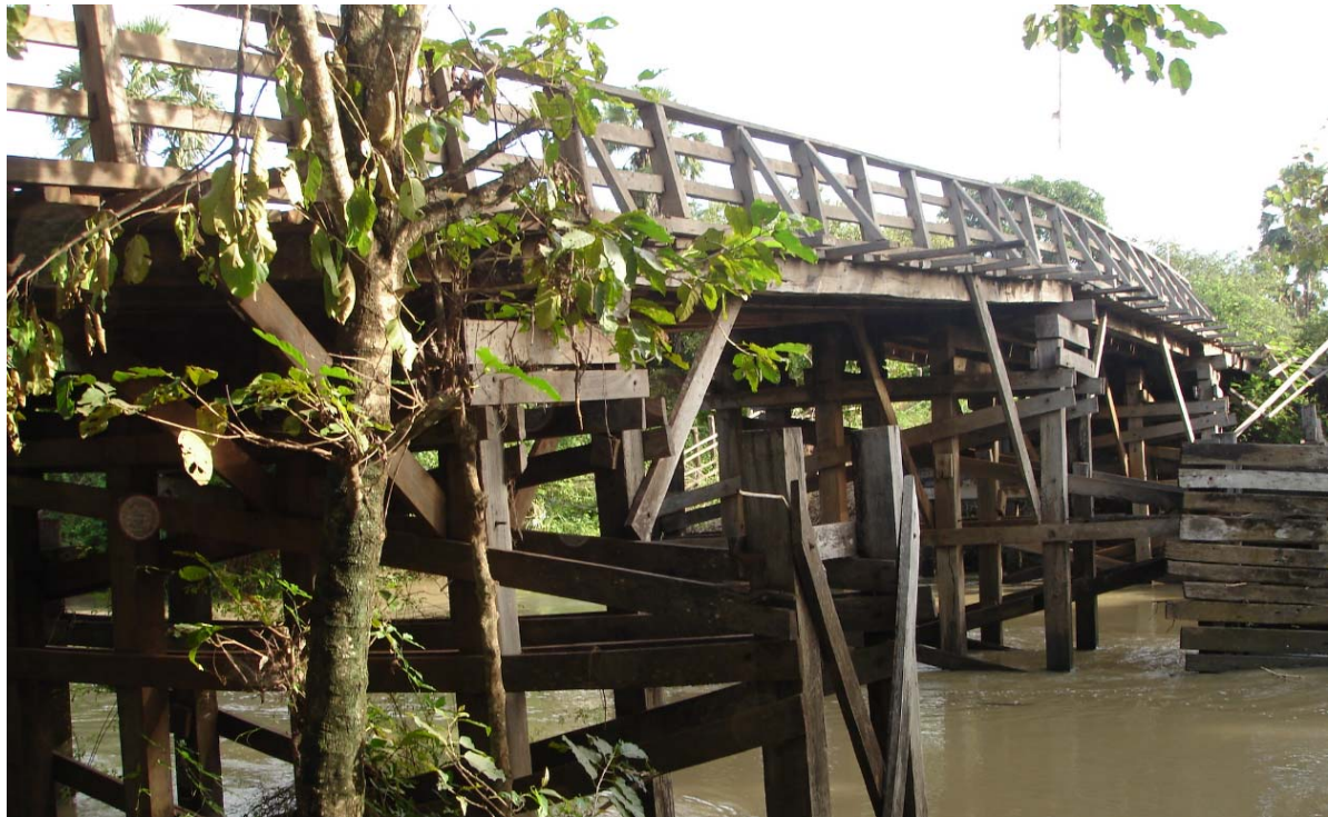
Existing O'trolouk Wooden Bridge at R213 Sta 2+ 559 (Preah Vihear)
