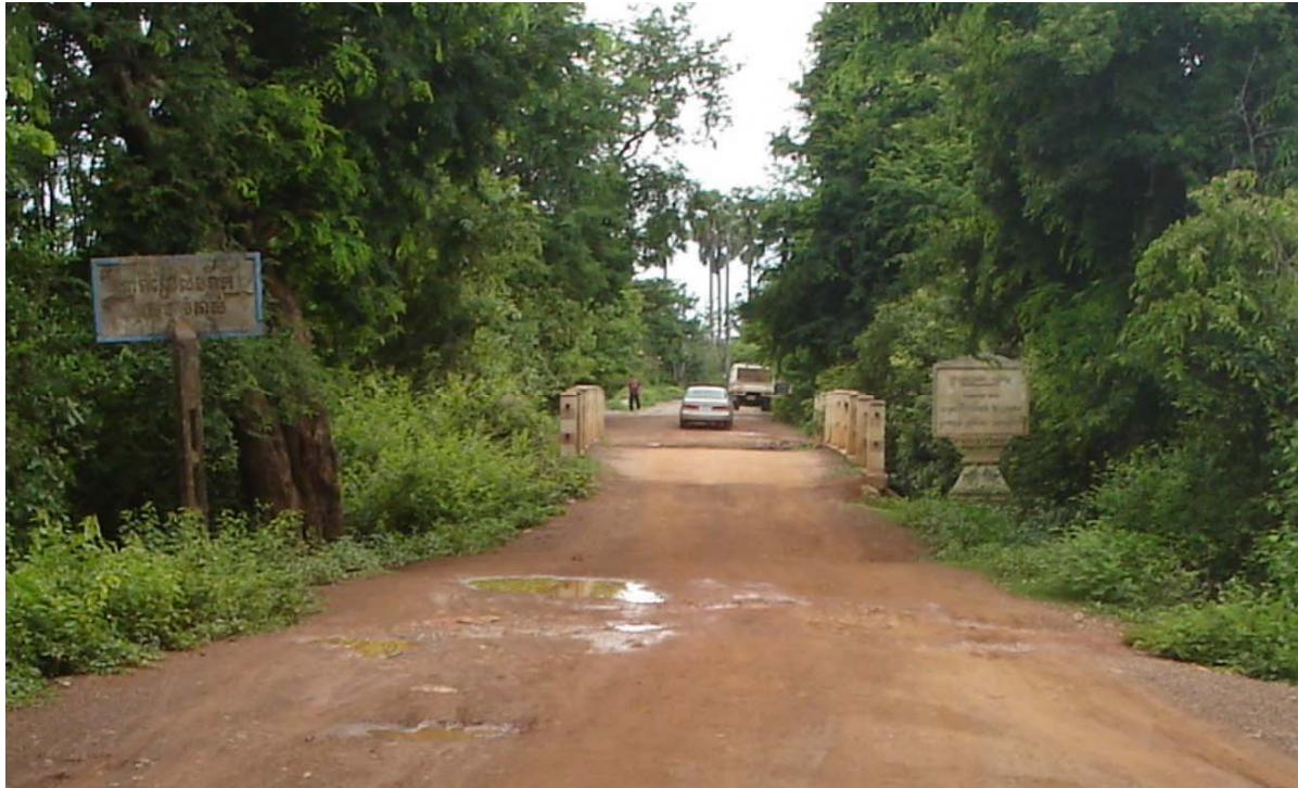
Existing Single Lane RC Bridge at PR207 (Siem Reap)
