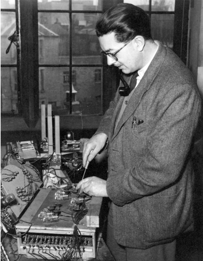
Figure 4: 'This apparatus had little lights, which were fixed with pins to the circular cork mat. The keys are morse code keys. One had to learn the position of each light (which was randomized) for each finger key, until the response was fast and automatic. Then the number of lights – that is the number of choices – was varied from 1 to 10. Reaction time was measured and integrated (with a mechanical integrator that W E Hick [left] made himself). The result was that the response time increased to the logarithm base 2, +1. This is called Hick's Law, which predicts the increased time a human will take to react to a stimulus as the number of possibilities increases. He attributed the number 1 to the choice of not pressing a key.' Professor Richard Gregory, 5 December 2002.
