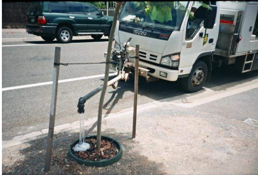
A street tree being watered with a Council water truck in Australia—note the product installed around the tree base for the purpose of delivering all the water applied direct into the tree root zone.
