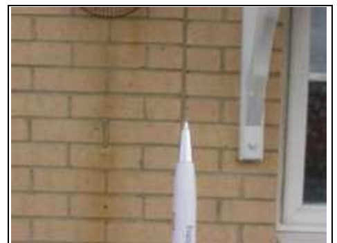
Mastic joint between two buildings
