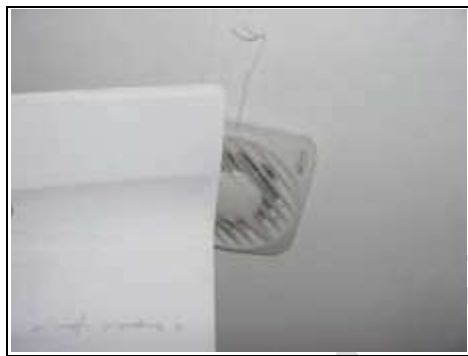
Extract system not working - Testing suction of extract fan by putting some paper against it
