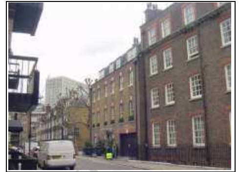
Older style London converted flats with property problems such as Condensation and Cold Bridging
