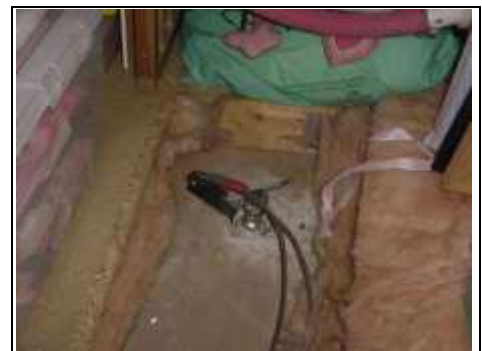
Ceiling lights cannot be covered
