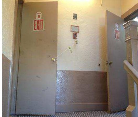
Fire doors illegally suspended open
