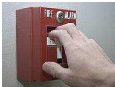
Activating a single action station
