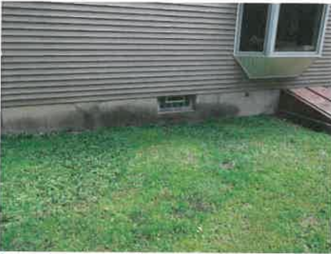
Area of negative grading above basement staining
