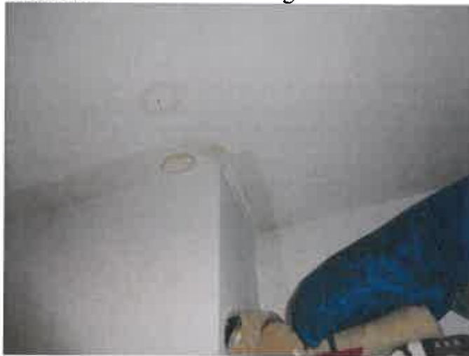
Water stain on second floor ceiling
