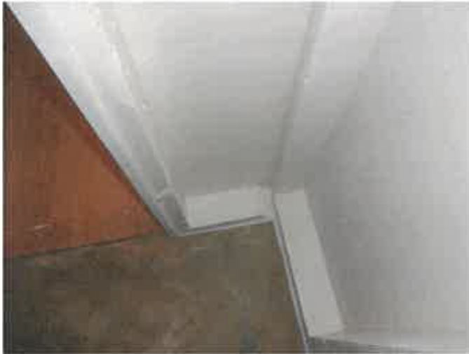
Gap between sill plates in corner has been painted
