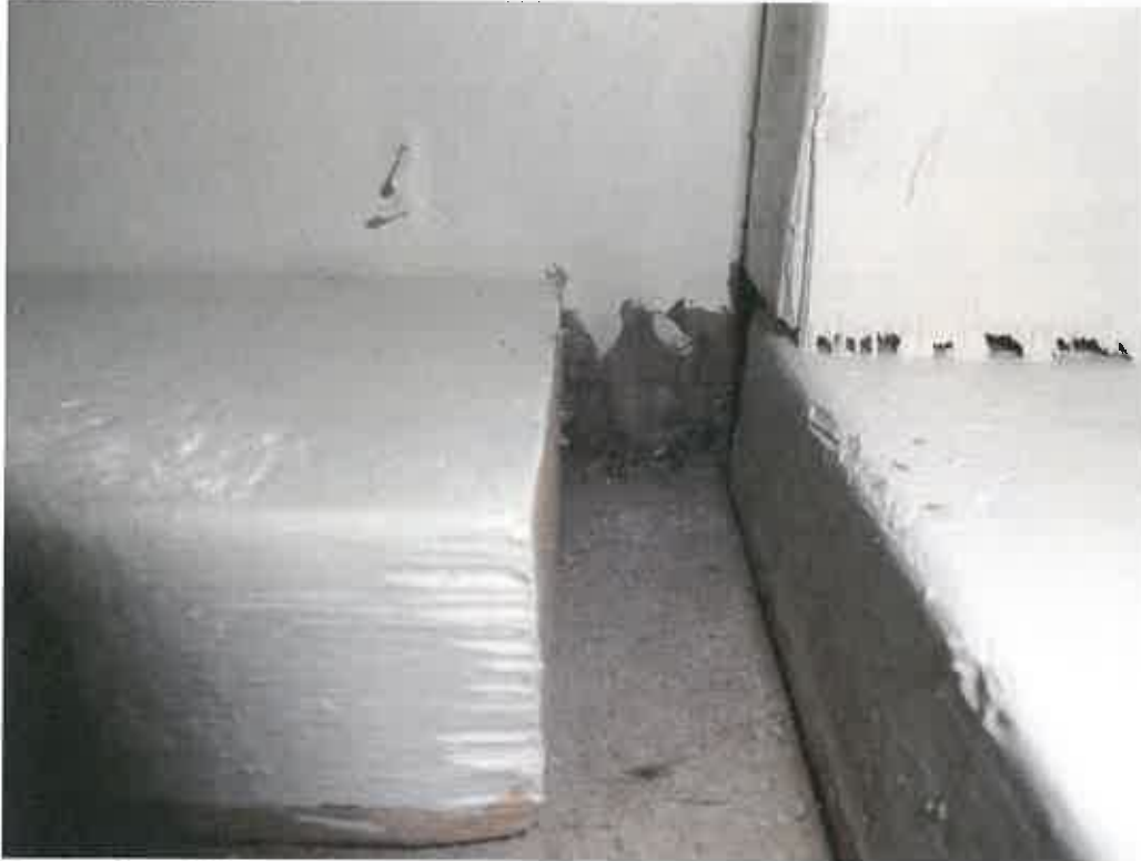
Sheetrock wall between 2x4's covered with Stachybotrys -close up view
