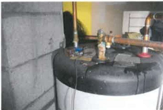
29. Water Heater: Tankless Coil-Integral w/ Boiler
