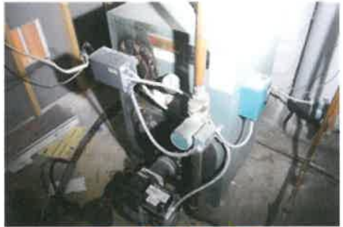
28. Heating System: Hydronic Boiler
