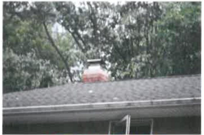
8. Roof Surface: Asphalt Shingle, Main roof
