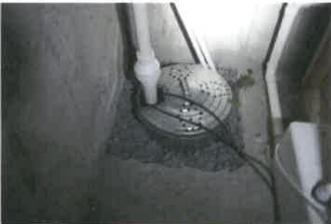
21. BASEMENT Sump Pump
