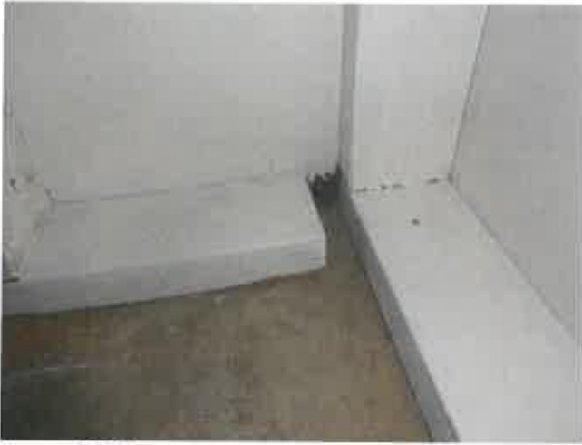
Area with Stachybotrys is between 2x4's
