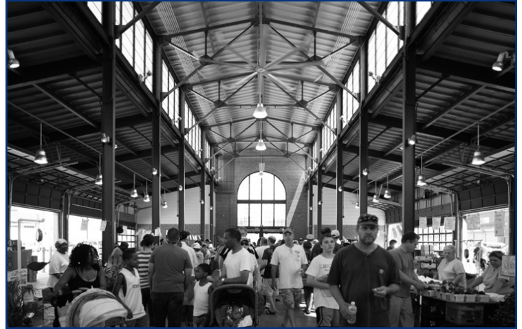
---explore the offerings at Eastern Market (courtesy of Christopher Lark Photography/Kraemer Design Group)...
