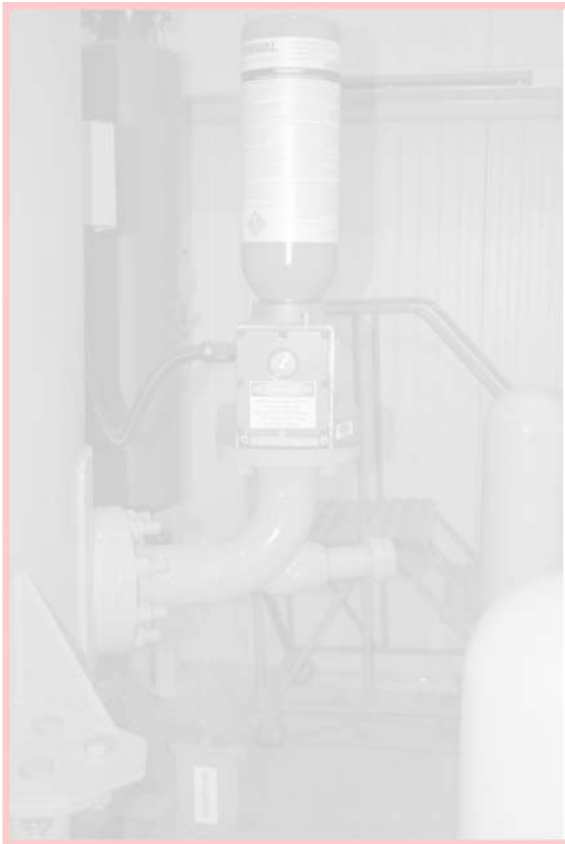
Figure 6.2.3.6.3(b) HRD Suppressor with Dual 20 mm HRD Valves.
