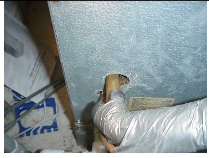
Exposed AC suction line, hall closet
