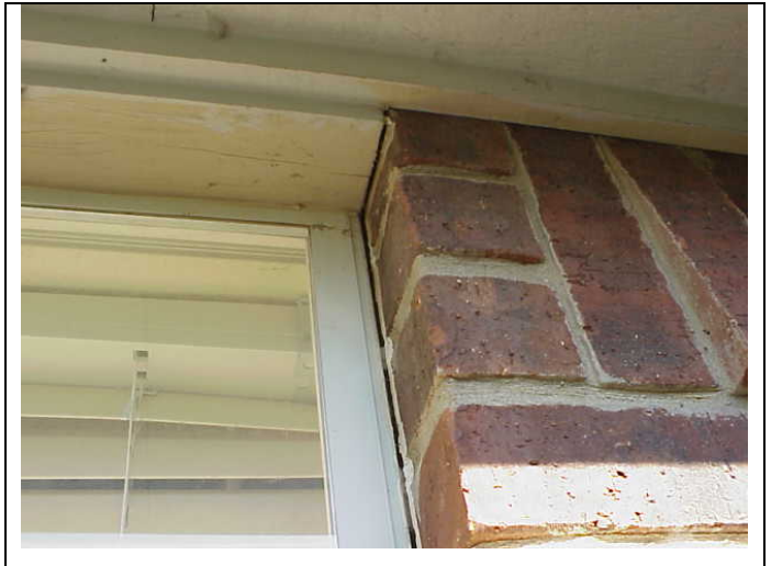
Separation of bedroom window frame, brickwork
