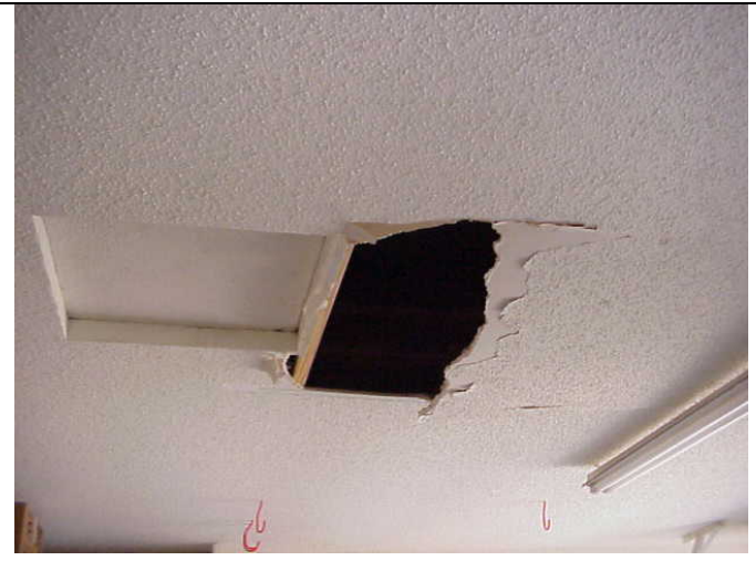
Hole in garage ceiling drywall
