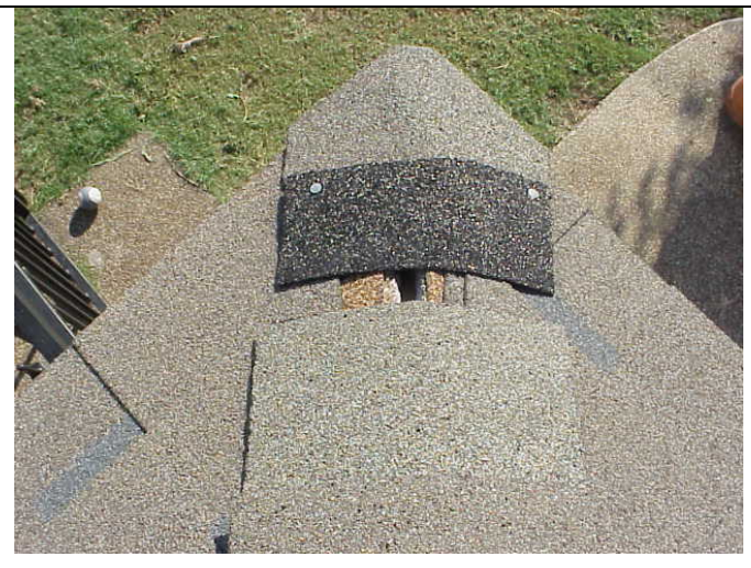
Ridge shingle missing, garage area
